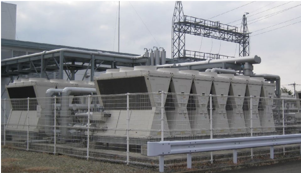
Heat pumps (Head Office Plant of Mochida Pharmaceutical Plant Co., Ltd.)
