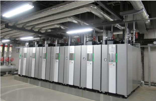
Gas-fired once-through boilers (Head Office Plant of Mochida Pharmaceutical Plant Co., Ltd.)
