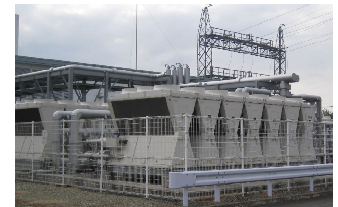
Heat pumps (Head Office Plant of Mochida Pharmaceutical Plant Co., Ltd.)
