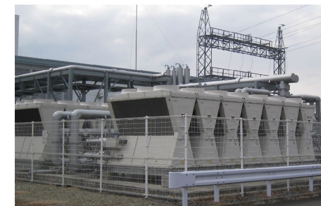
Heat pumps (Head Office Plant of Mochida Pharmaceutical Plant Co., Ltd.)
