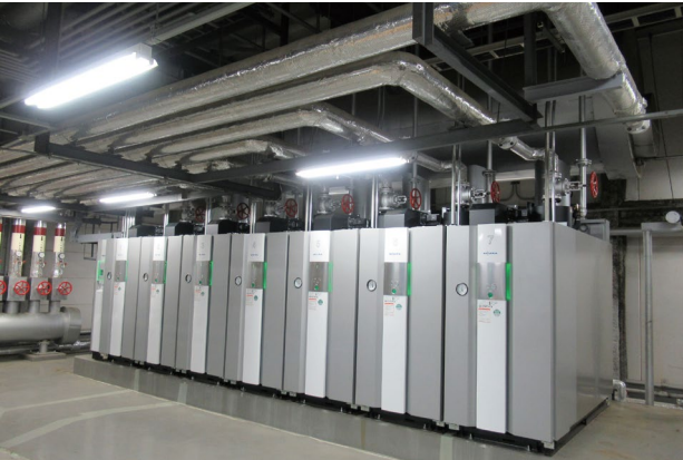
Gas-fired once-through boilers (Head Office Plant of Mochida Pharmaceutical Plant Co., Ltd.)
