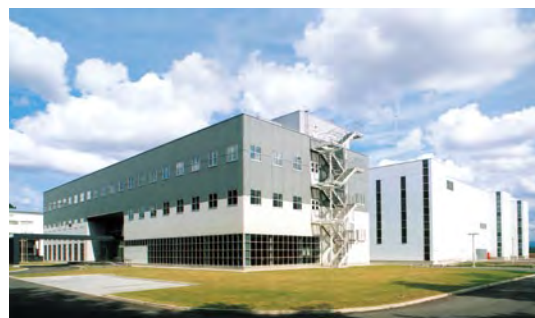
Mochida Pharmaceutical Plant Co., Ltd. Head Office Plant
